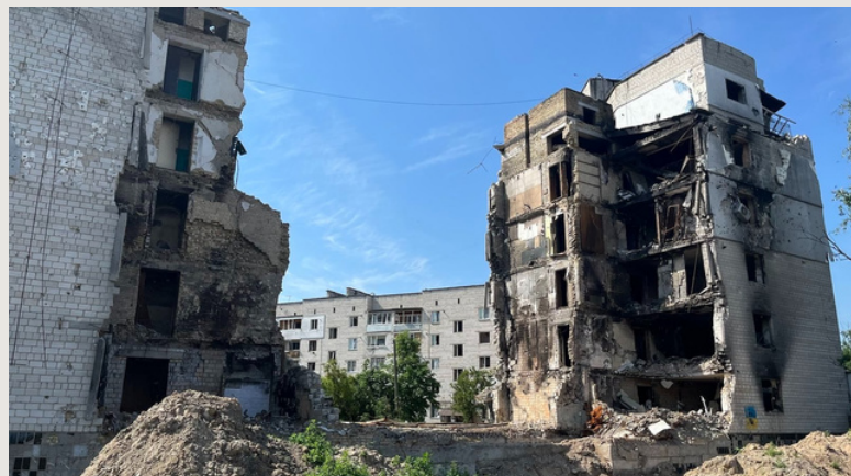
Destroyed by Russian aviation apartment buildings in Borodyanka, Kyiv region.
